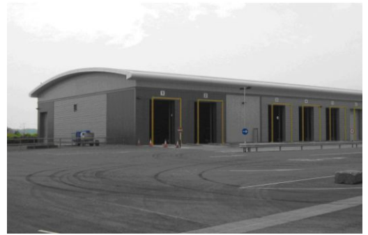
Built form of Alconbury Waste Transfer Station
