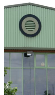
Ventilation should be incorporated into facade design
