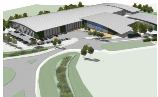
A good example of built form
