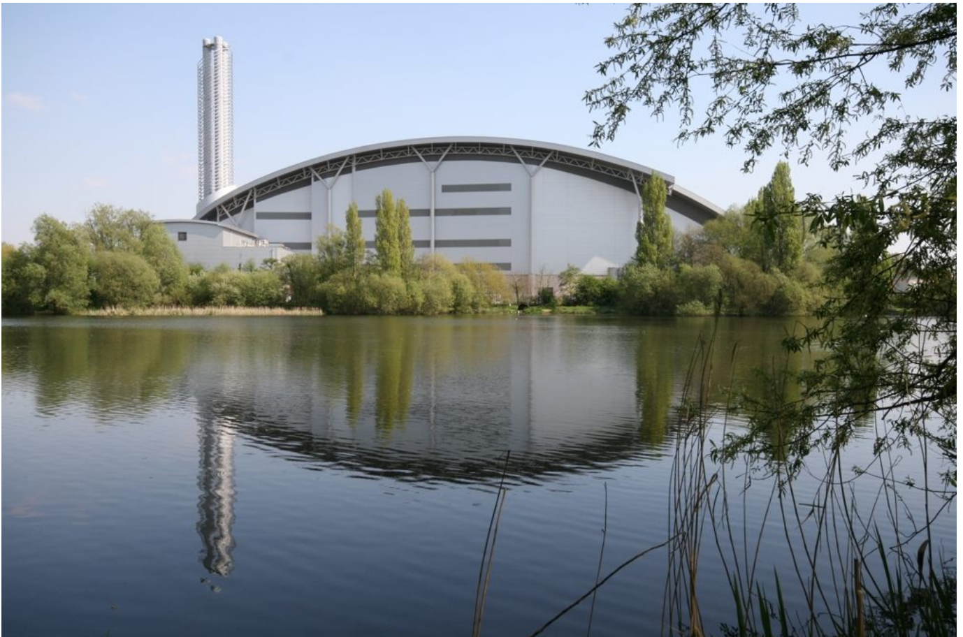
Energy from Waste Facility Lakeside (Grundon)
